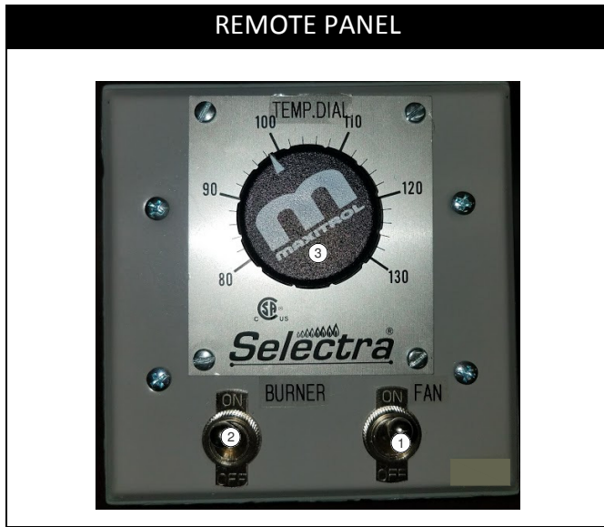
FIGURE 16.1 - TYPICAL REMOTE MONITORING (MAXITROL 14 SHOWN)
